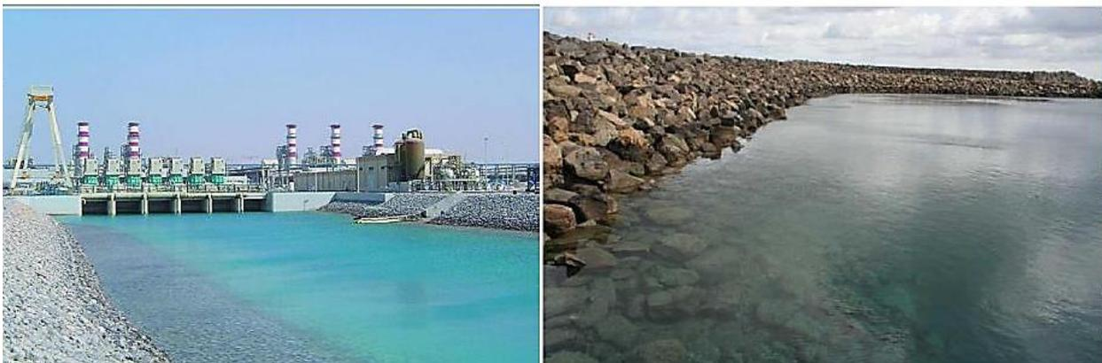
Figure 6: Examples of open intake basin protected by breakwaters (Andries *et al.*, 2014)
