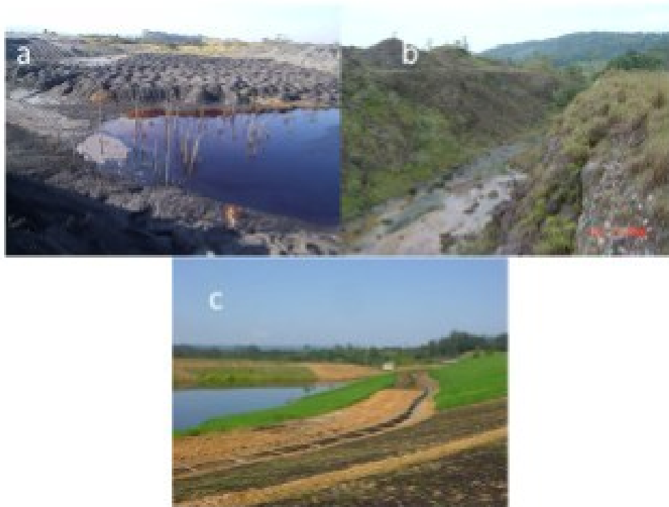
Fig. 1. a: Coal waste and an acidic pond, b: Surface mined area and spontaneous vegetation, c: Clay cover, spread soil, and vegetation [6].
