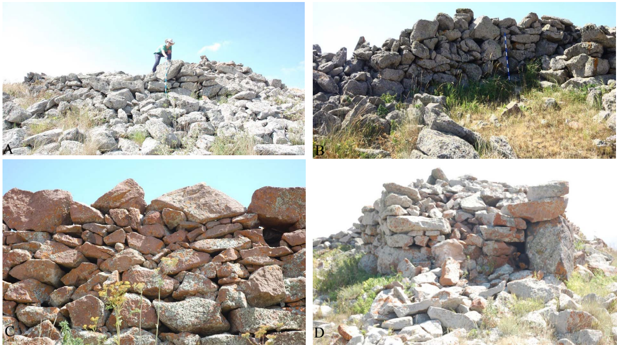
Figure 10: Different views of photographs showcasing wall construction techniques (a-d) (Photo by A. Ceylan 2013).
