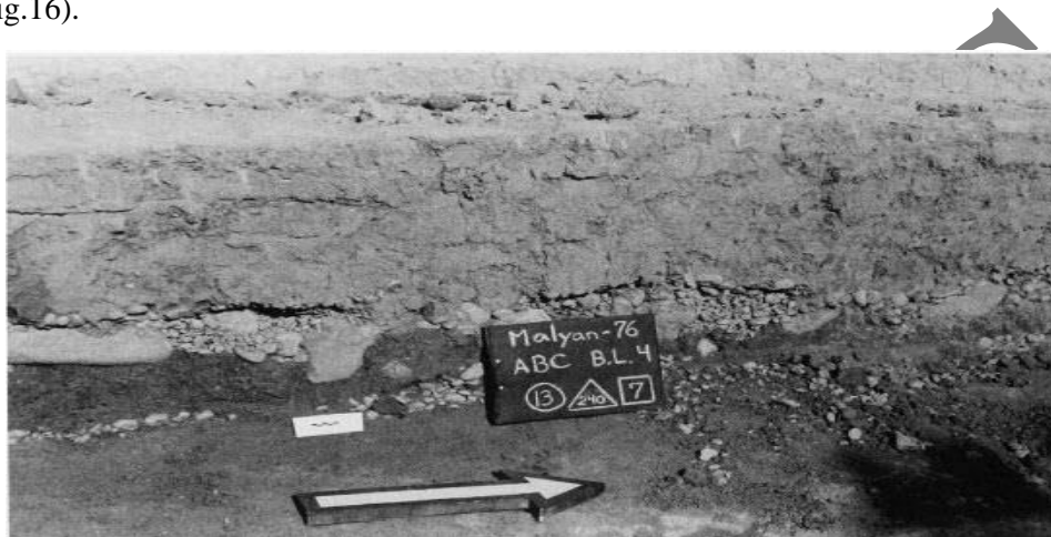
Figure 16: Coarse-grained sediments utilised in the foundation of structures at the ABC operation (After: Sumner, 2003: 340)
